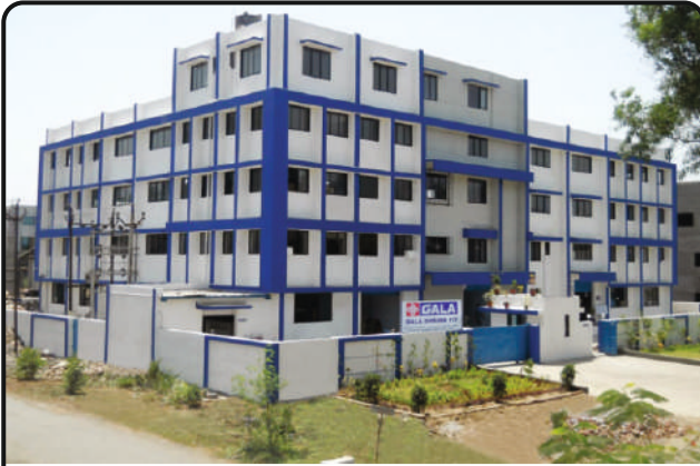
UNIT - 2 Moulded Shape Factory - Surat
